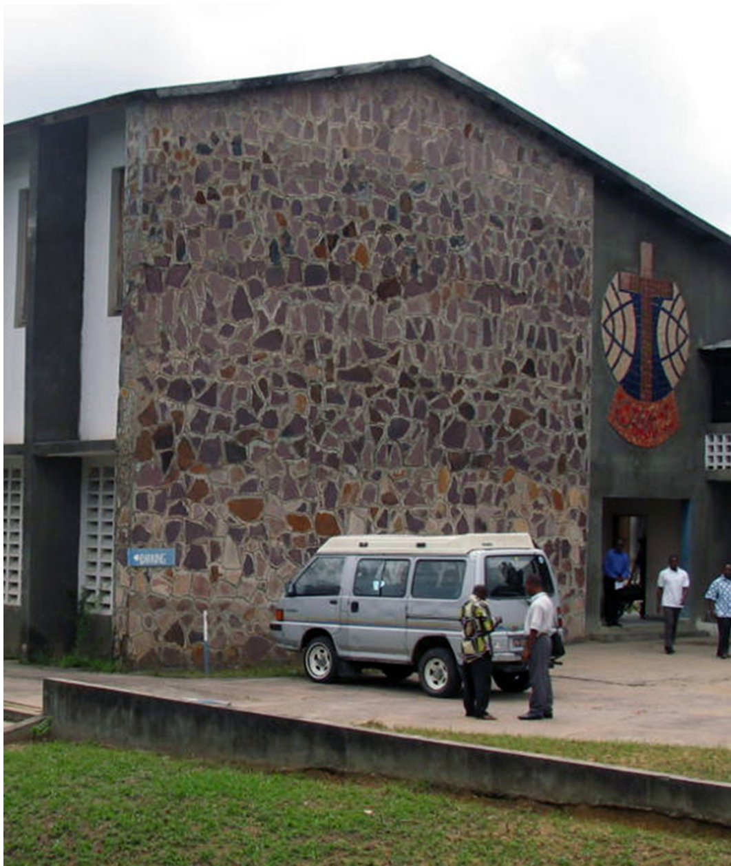
Fig. 4 - Example of facade with Cretaceous sandstone slabs, Faculty of Mazenod, apse of the chapel. On this facade veneer of the building was found the slab Kin 03.
