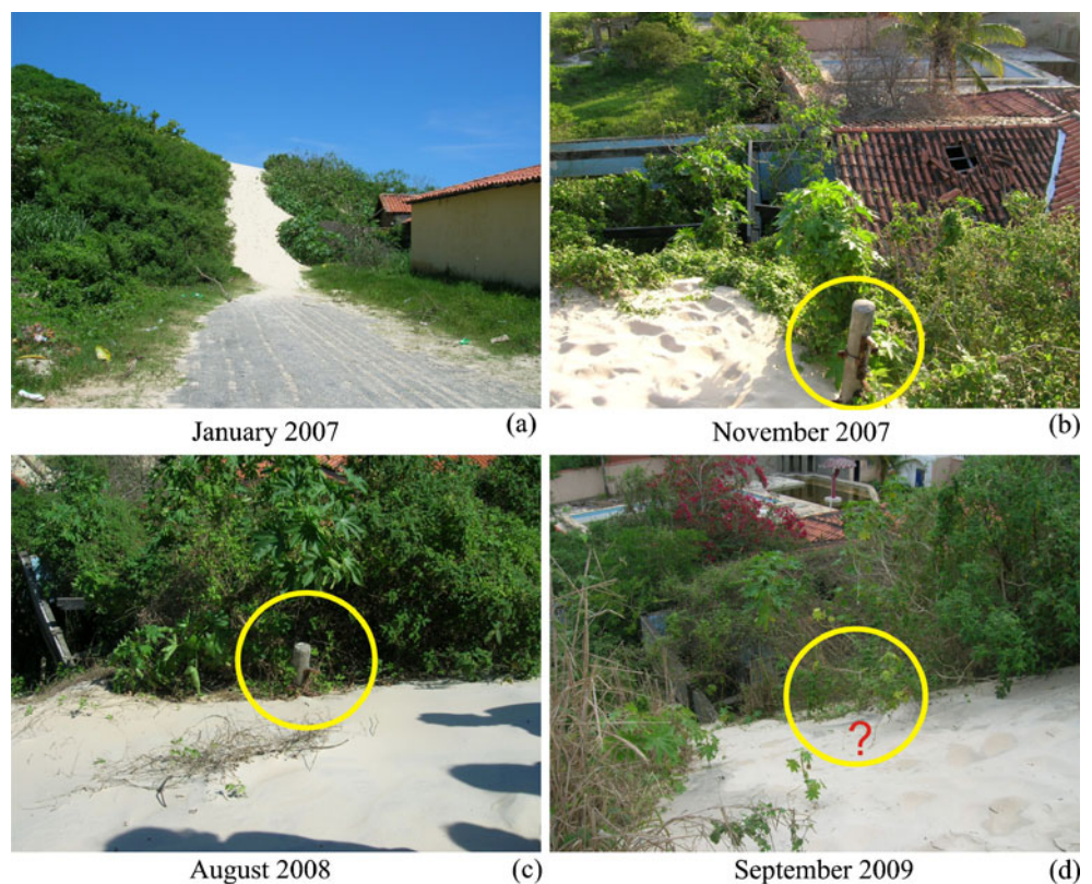
Fig. 8 Geological risk associated with the Perú dune field. The construction of houses/building in the direction of the dunes' movement reveals the consequences of occupation without any prior technical risk evaluation. b, c, d Successive engulfment of a lamp post by sand (encircled)
