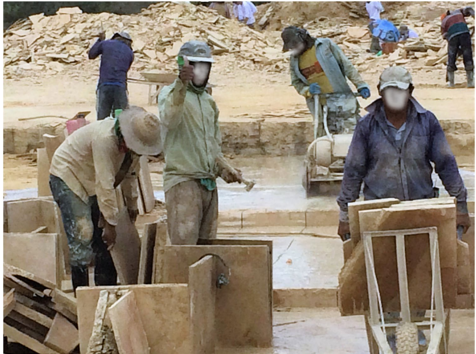
Fig. 3 Quarry in the Araripe Basin, in Brazil, where slabs of rocks are produced for construction and industrial use. The discovery of fossils by laymen is common on this and other mining fronts throughout Brazil. However, the names of the workers involved in the discoveries are deliberately omitted, either as a form of protection against possible criminalization of the discovery, or the lack of intellectual integrity of researchers who constructs a narrative in which the reality of discovery is only seen from their own creation. Blurred faces to prevent any kind of judicial retaliation by paleontologists who work in the region of the Araripe Basin and linked to federal and state public institutions
